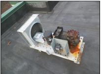
**E.** (2) Both Domino's Pizza and Silk Road Bistro contained large exhaust hoods over the oven and range areas. Observed connected roof-top exhaust fans. Captiveaire commercial kitchen ventilation system equipment appeared to be of recent age and was operating during the inspection. An older Aerolater (Captiveaire systems) exhaust unit was observed at the north portion of the roof with a serial #II-36818 and 2,000 cfm rating.
