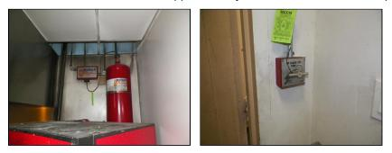
**B.** Fire alarm pull station for the bistro space and portable fire extinguishers were observed through the 2 visited tenant spaces. The fire suppression alarm system appeared to be operable.
