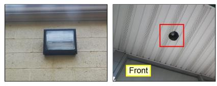
**I.** Building was equipped with battered-powered "frog eyes" emergency light fixtures throughout the inspected tenant a and b spaces. They appeared to be sufficient in number and location as to properly facilitate emergency excavation.
