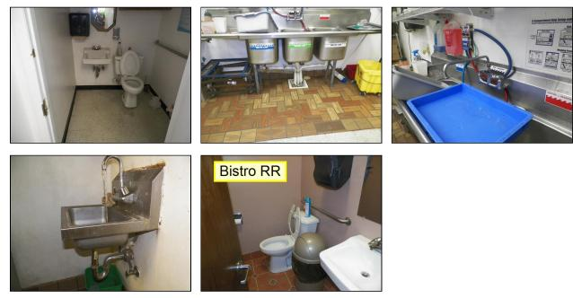
**B.** (1) Observed drain plumbing and traps underneath restroom and kitchen sinks. Tenant a (Domino's Pizza) had at least two plumbing leaks between pvc fixtures.
