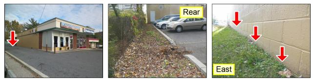
**B.** It appeared that the property had a peak elevation near the northwest corner of the building. All pavement to the south drained by sheet flow onto Smith Road to storm drain inlets near Main Road and eventually discharges into a Baltimore County 36" storm drain main along Main Road. Pavement to the north, basically the rear parking lot, drains in an easterly direction to two curb cuts that discharge the storm water onto grassy area of the golf course property.
