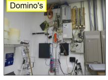
**G.** (3) The electrical distribution shut-off Cutler Hammer boxes and their connections were severely deteriorated at least 3 RTUs. Recommend replacement.
