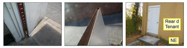
**F.** The masonry walls extended past the roof surface elevation and formed a perimeter parapet wall. The wall's top surface was covered by sheet metal coping. Observed openings in the overlapping pieces of the coping material, exposed fasteners and mastic material. Mastic deteriorates and shrinks over time thus causing potential openings hence water intrusion possible locations. Recommend the roof installer be contacted to seal openings/nail heads and other necessary items.
