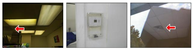
**E.** (1) See 5.D for roof-top cooling equipment including Lennox, Carrier, York and Fraser-Johnson units. These cooling units provided cooled supply and return air throughout the interior spaces through large metal ductwork to ceiling diffusers.
